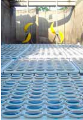
Combining aeration & mixing technologies
