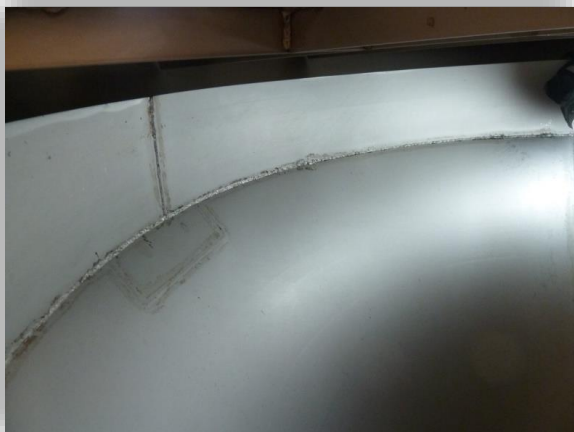
Overflow weir for the continuous discharge of the liquid phase
