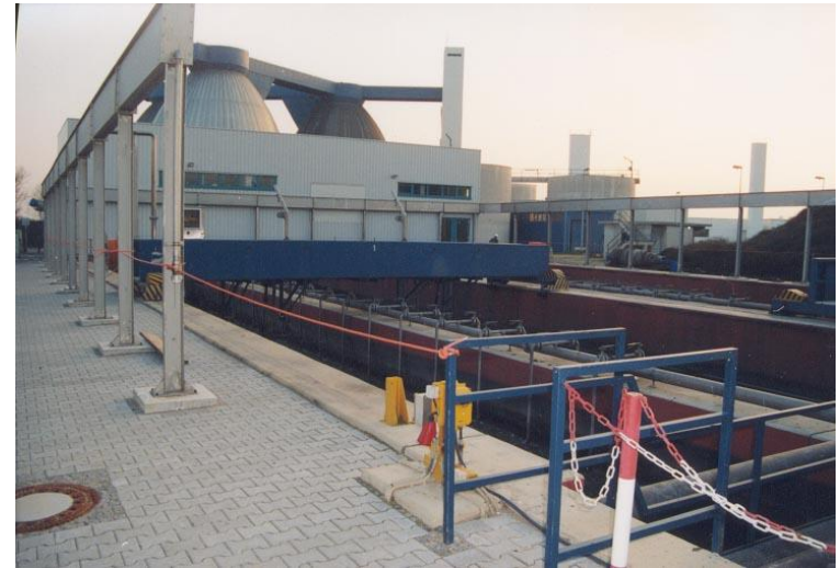
Grit trap on WWTP Mannheim
