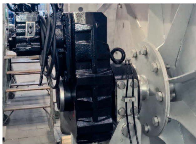
Low-maintenance chain drive on the HUBER Drum Screen LIQUID
