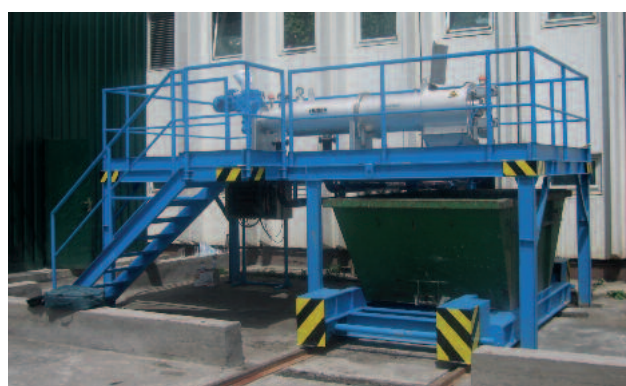
Outdoor installation of a HUBER Sludgecleaner STRAINPRESS®
