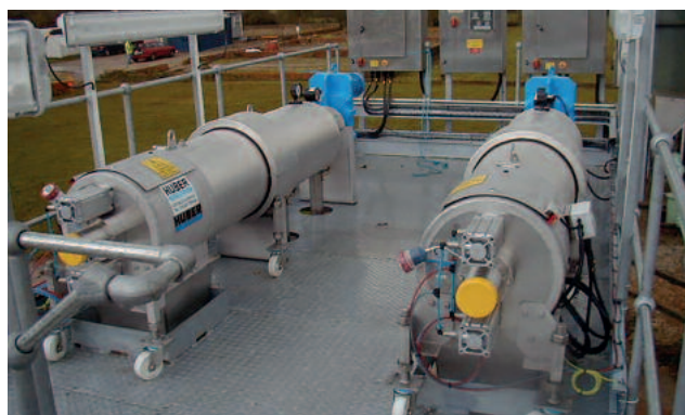
STRAINPRESS® with heatable casing pipe
