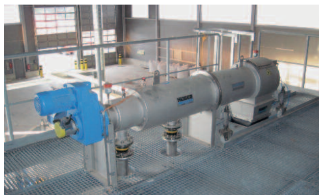
Screen for the removal of fermentation residues
