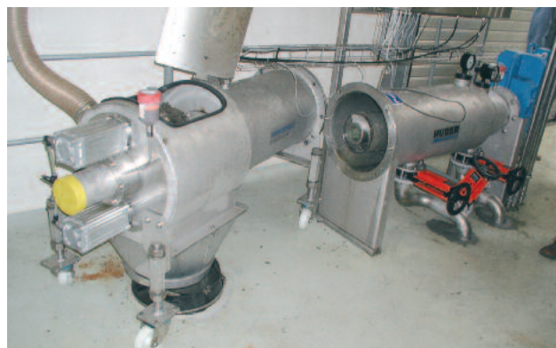
Splittable casing
