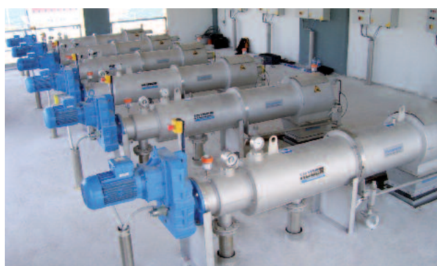
Sludge screening on WWTP Athens, Greece
