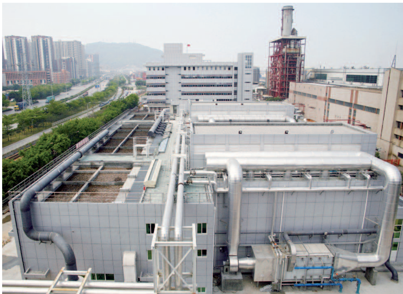
Large-scale sewage sludge drying plant with external condensation units and biofilters
