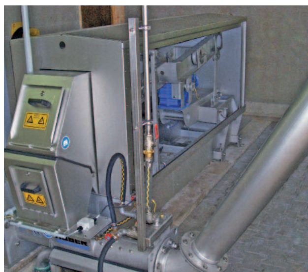
Channel installation of a HUBER Curved Bar Screen CurveMax® with downstream wash press
