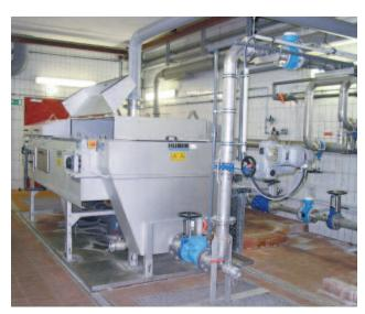
Belt thickener for 60 m<sup>3</sup> thin sludge per hour
