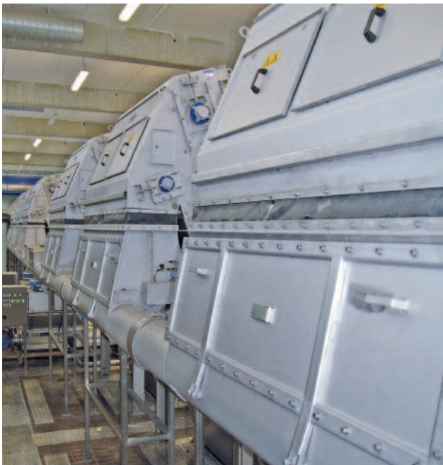
Rear view of the HUBER Belt Screen EscaMax® with subsequent laundry channel for wear-free screenings transport
