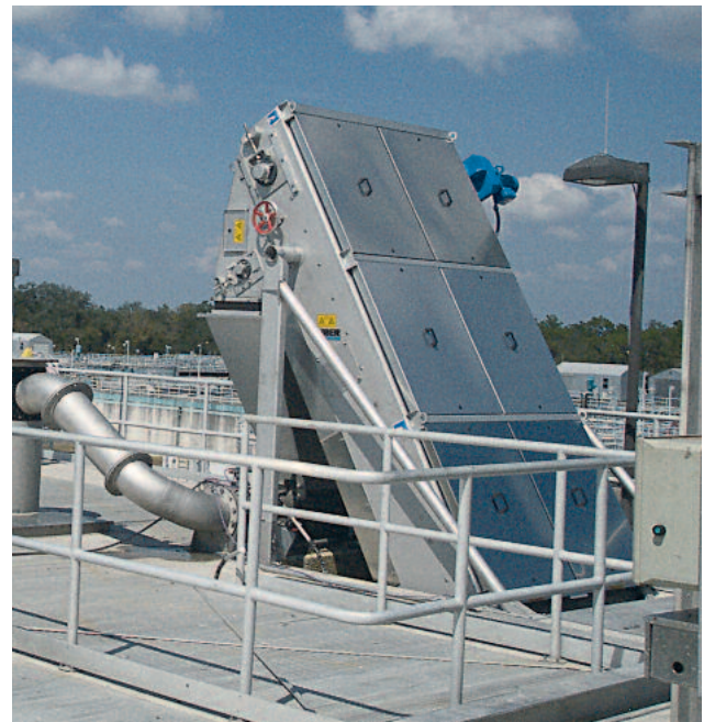
Fully enclosed, odour-free screen with easy to remove covers
