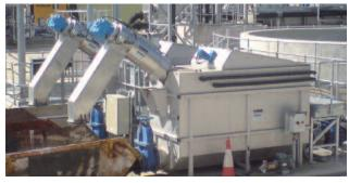
ROTAMAT® Membrane Screen RoMem units in tanks
