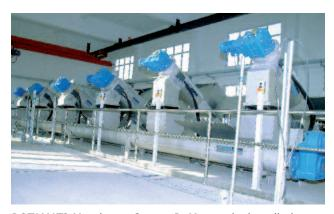
ROTAMAT® Membrane Screen RoMem units installed to protect a large downstream MBR plant
