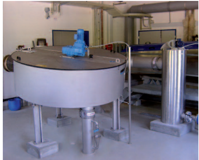
ROTAMAT® Disc Thickener RoS 2S size 2 with preceding flocculation reactor
