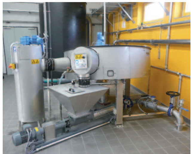
ROTAMAT® Disc Thickener RoS 2S designed to thicken 35 m 3 /h
