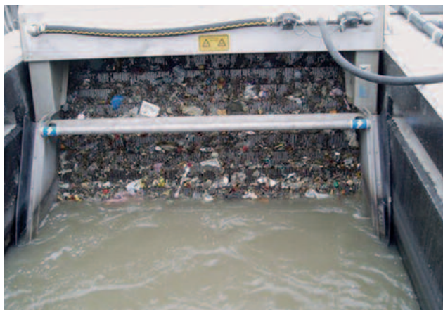
STEP SCREEN® Flexible SSF: length 3500 mm, width 1826 mm, 6 mm slot width, 50° installation angle. High capacity as the flow passes the screen surface only once.
